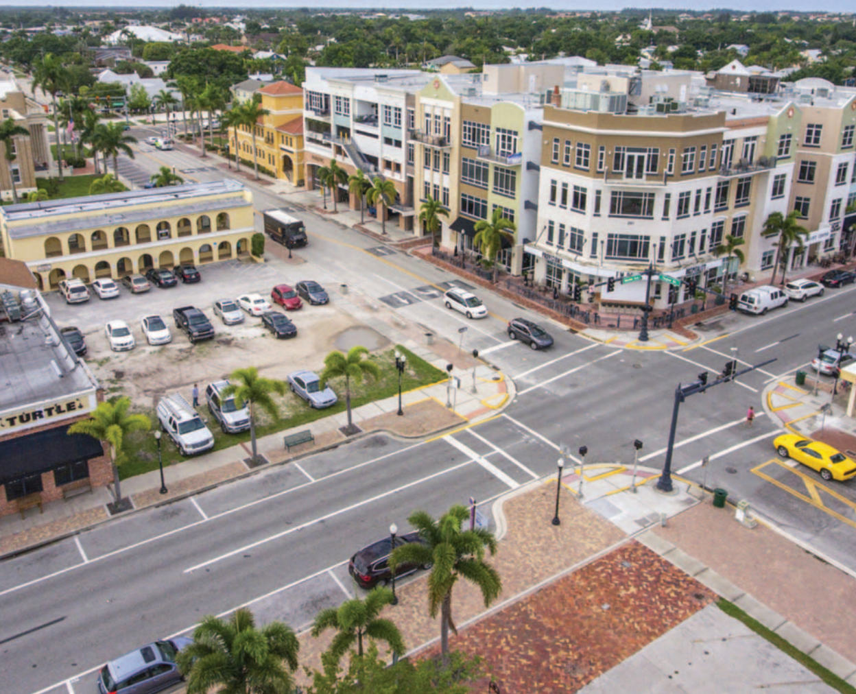
Aerial photo of intersection of Marion Avenue and Taylor Road in downtown Punta Gorda.
